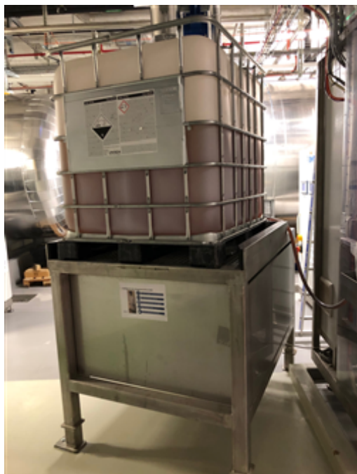
IBC RO - with containment.jpeg
