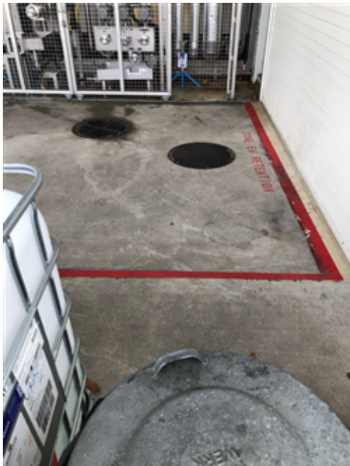
unloading area with retention zone.jpeg
