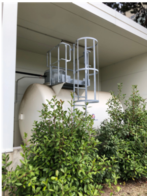
Diesel tank.jpeg
