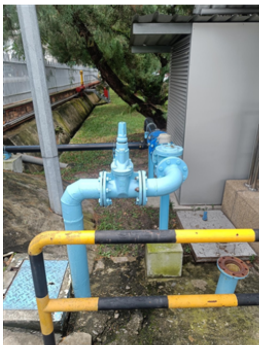
Water incoming to site pipeline and meter (air selangor meter).jpg
