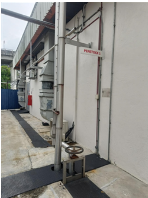
Penstock Valve to contain any potential chemical spill.jpg
