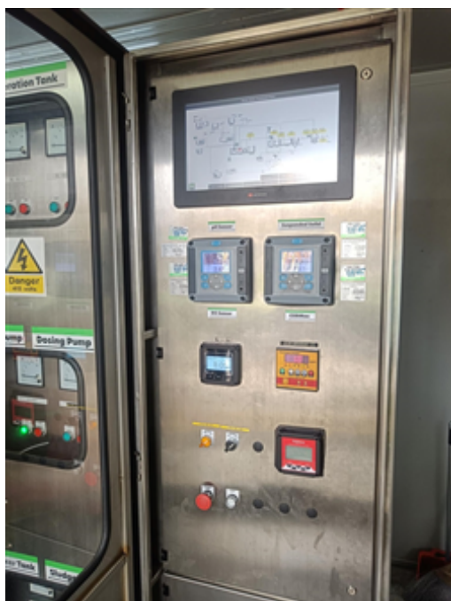
SCADA system with inline monitoring sensor for Wastewater effluent.jpg
