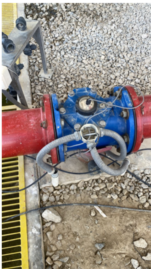
Each irrigation line has its own flowmeter Batch C5 PHOTO-2024-10-16-12-16-02.jpg
