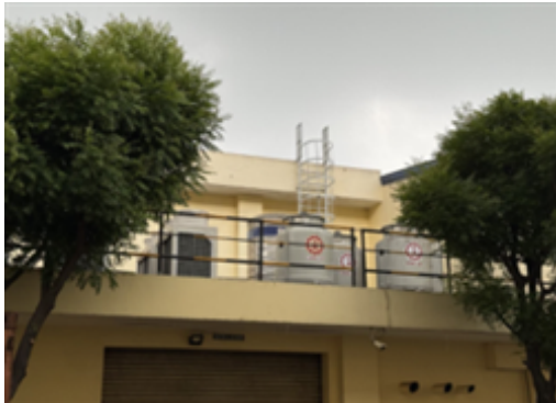
2m3 inox tank on the roof used for cooling tower.png
