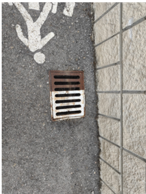
Grating for collecting rainwater.jpg
