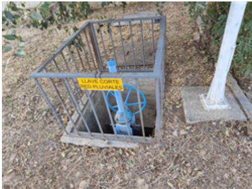
Rainwater shut-off valve.jpg
