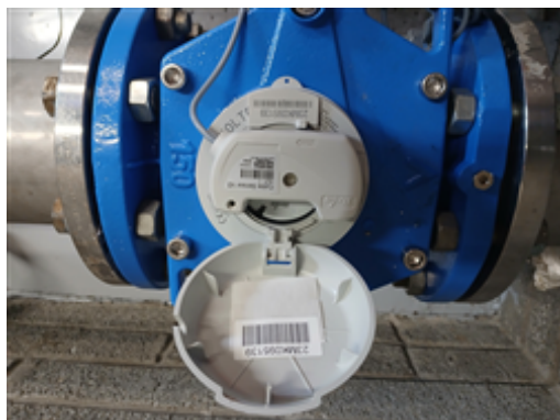
07 OC Water Meter in Chlorine pump house.jpg
