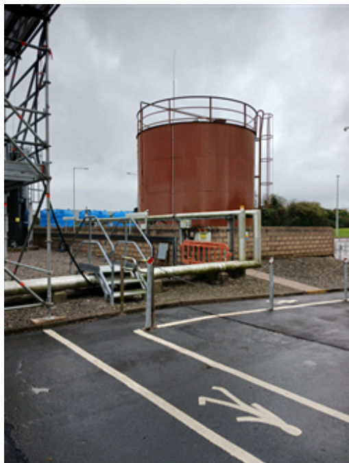
60 OTC Diesel Tank for Boiler.jpg
