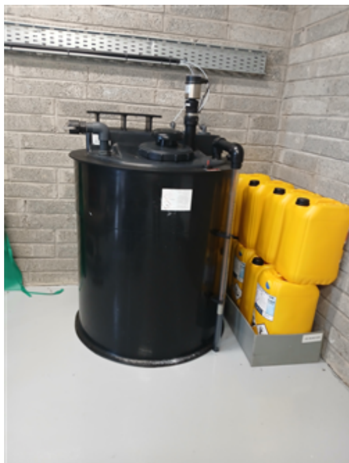
08 OC Chlorination Tank and Chemical Bund.jpg
