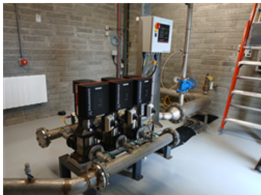
04 OC Process Water Pumps.jpg
