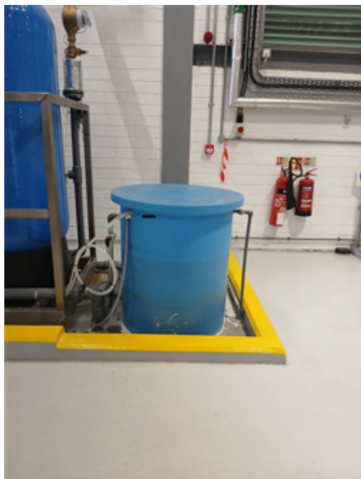
31 Biomass Water Softening Tank.jpg
