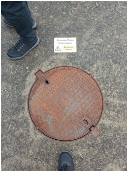
14 OC Process Drain Interceptor.jpg
