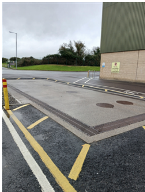
61 OTC Diesel Delivery Point with spill protection.jpg
