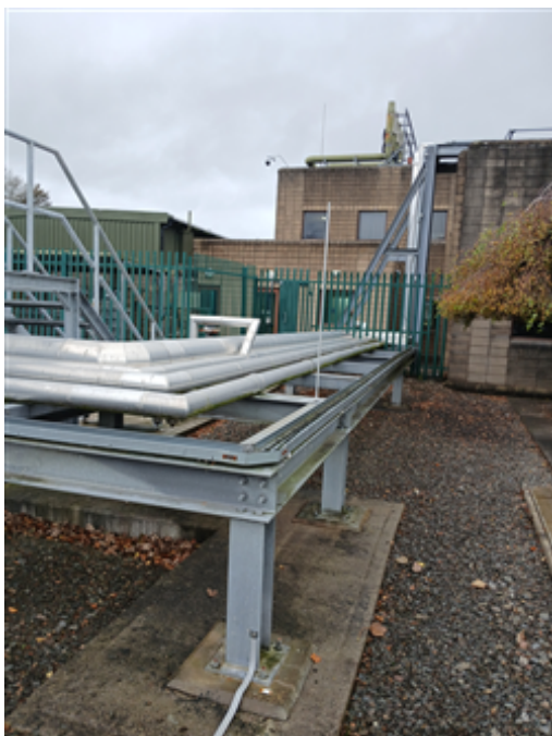
56 OTC Steam pipe from Biomass.jpg
