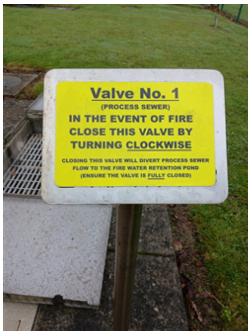
16 OC Stormwater Pollution Bypass Valve to Retention Pond.jpg
