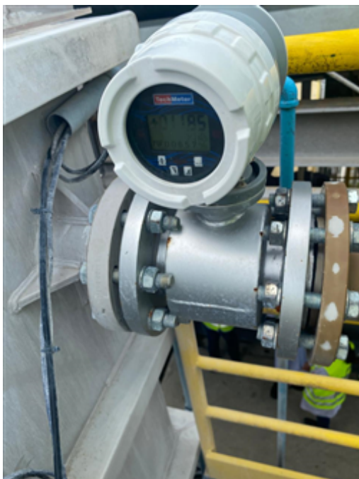
6. IWTP - Lamellar decanter - flowmeter.jpeg
