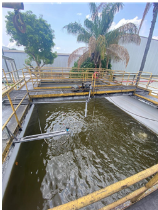
6. IWTP - CT15 - Equalization tank1.jpeg
