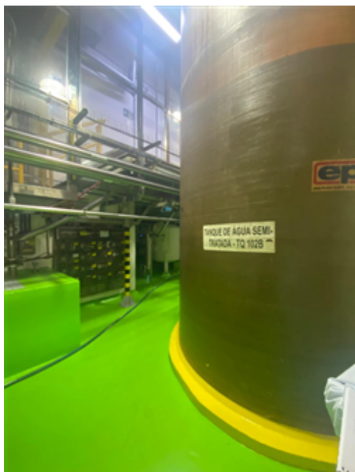
3.WTP - Semi-treated tank.jpeg
