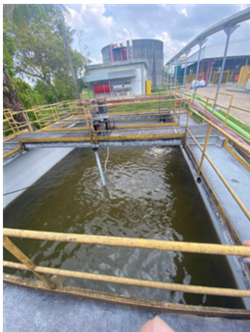
6. IWTP - CT15 - Equalization tank.jpeg
