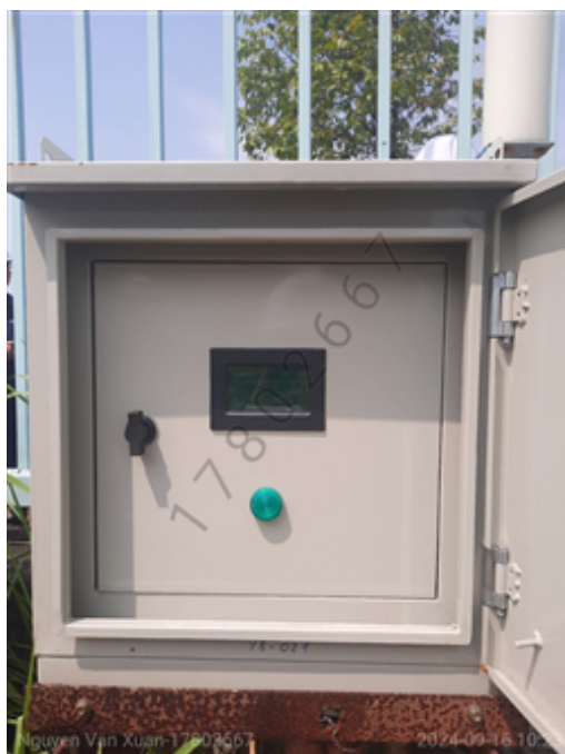
SEVT1 Supply water flowmeter indicator line 3.jpg
