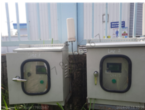
SEVT1 Supply water flowmeter Line 1.2 indicator.jpg
