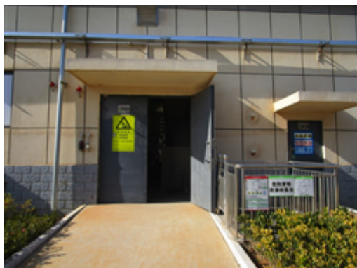
Hazardous waste storage area.JPG
