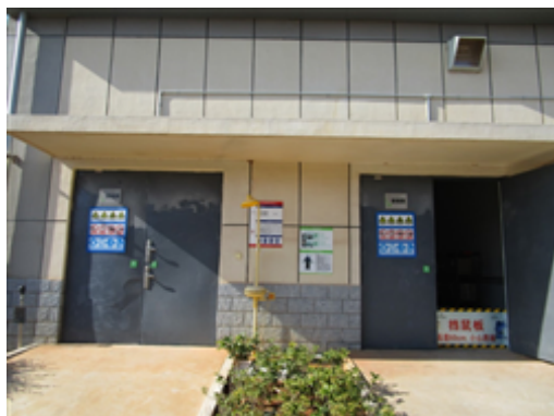
Chemical storage area-2.JPG
