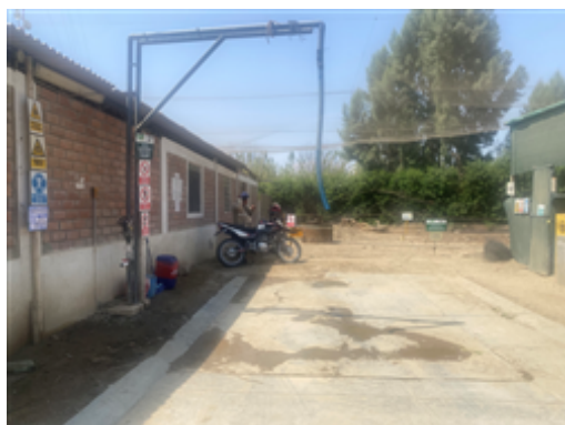
Water supply for fumigation machines - Don César Farm
