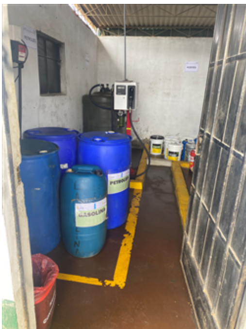
Fuel and oil storage - Guerrero farm. IMG_3282.jpg
