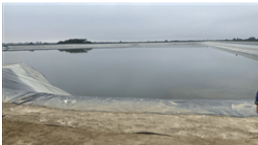
Fundo Don Guerrero: Reservoir with a capacity of 350,000 m³. WhatsApp Image 2024-11-17 at 16.53.32.jpeg
