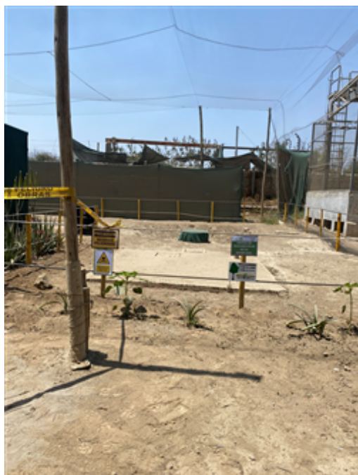
Wastewater Treatment System - Don Lito farm IMG_3659.jpg
