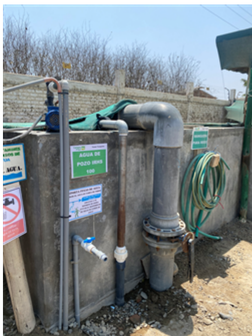
Water inflow to the pool of the IRHS 100 well at Tronquitos Farm
