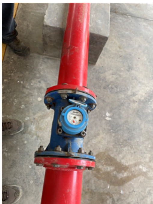
Flowmeter in irrigation and fertilization room at Tronquitos farm
