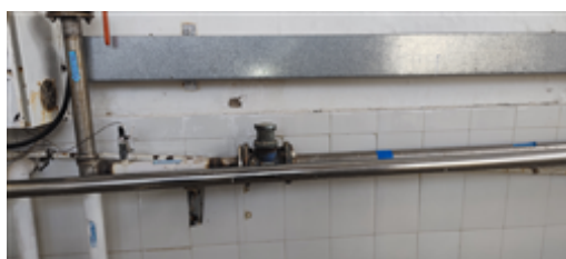
DM plant water flowmeter.jpg
