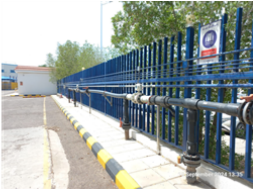
Site water inlet and flow meter.jpeg
