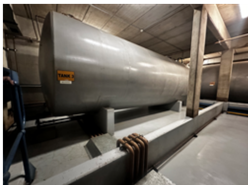
Diesel storage tank 3 with bunding.jpeg
