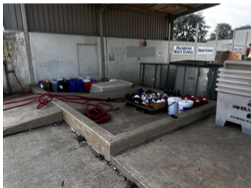
Bunded area for temporary storage of liquid waste in the Waste Handling Facility.jpeg
