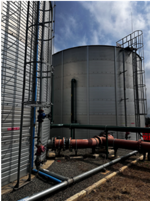
Site storage tanks and pipework.jpeg
