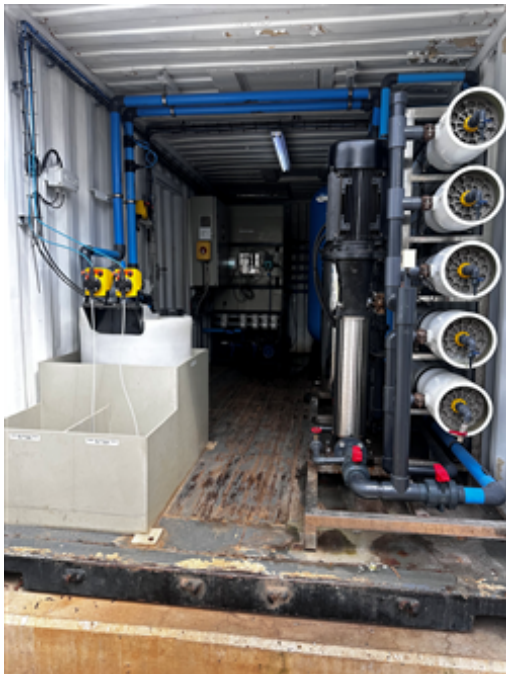
RO plant next to the site's storage tanks.jpeg
