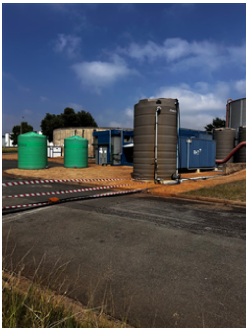
Site water storage tanks next to the first RO plant.jpeg
