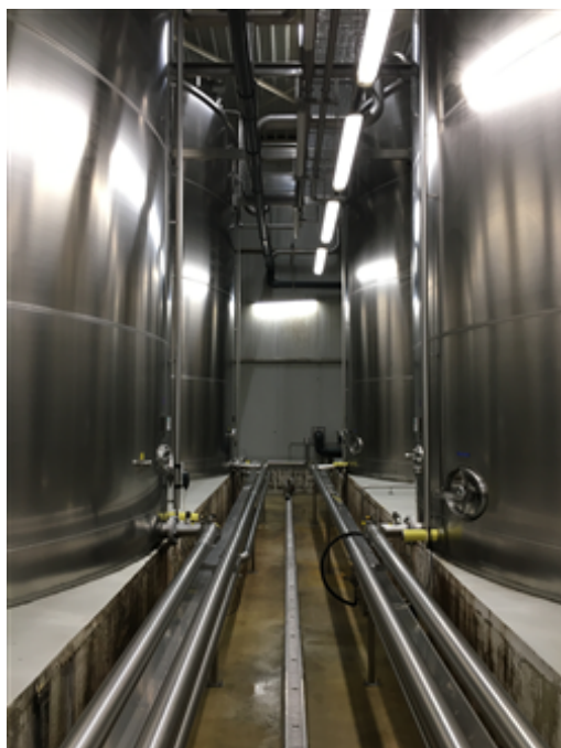
Photo 07 - 6 storage tanks of 160m3 each, to store water used in production and industrial processes (source Nestlé Waters Benelux).JPG
