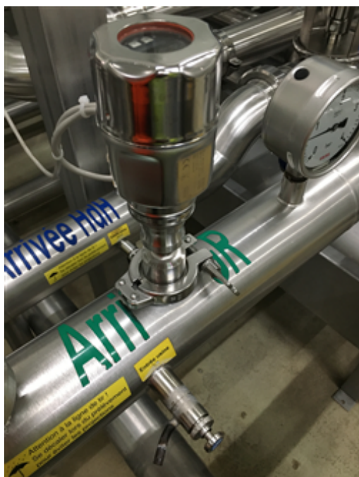
Photo 01 - Pipelines entering the factory (GR and HdH) (source Nestlé Waters Benelux).JPG
