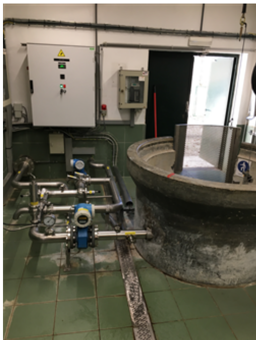
Photo 10 - Fond de Volette FDV wellhead, water sampling tap and flowmeter (source Nestlé Waters Benelux).JPG
