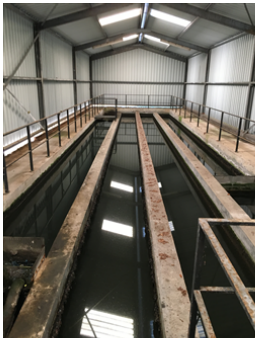
Photo 08 - Neutralization station, sedimentation basin (source Nestlé Waters Benelux).JPG
