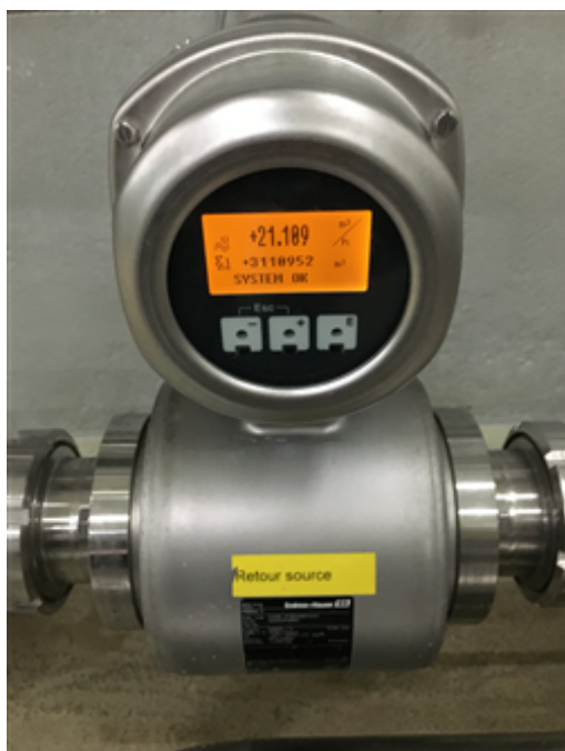
Photo 06 - Pipeline and associated flow meter for the “retour source”, returning unused water to the environment (loop) (source Nestlé Waters Benelux).JPG
