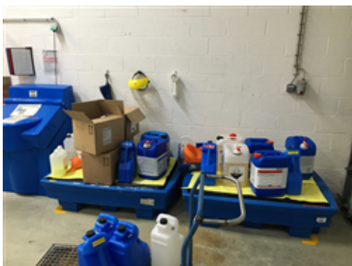
Photo 03 - Chemical product storage areas (acid and base) (source Nestlé Waters Benelux).JPG
