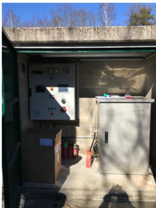
Photo 09 - Buffer pond area (pond isolation valve, sampling point, flow meter, continuous pH and temperature monitoring screen) (source Nestlé Waters Benelux).JPG
