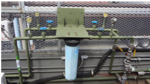
filter for the water from the mains.JPG
