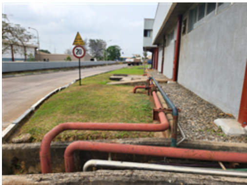
Firefight hydrant pipeline.jpg
