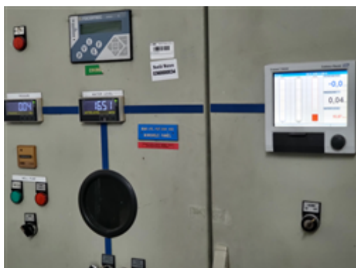
Borehole monitoring panel.jpg
