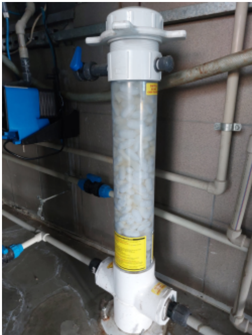
Chemical_dosing_system_for_water_treatment_in_cooling_towers.jpeg
