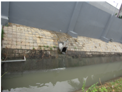
2. Storm water Outfall point.JPG
