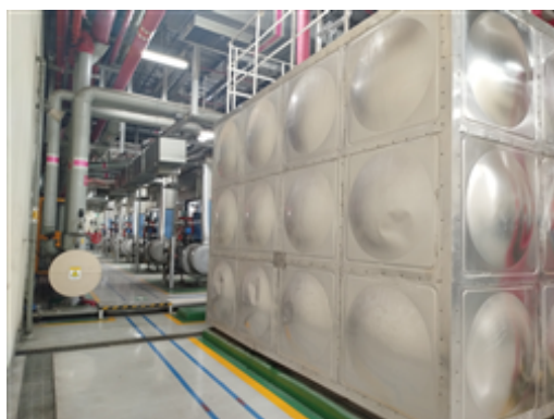
9. RO tank of Boiler .jpg
